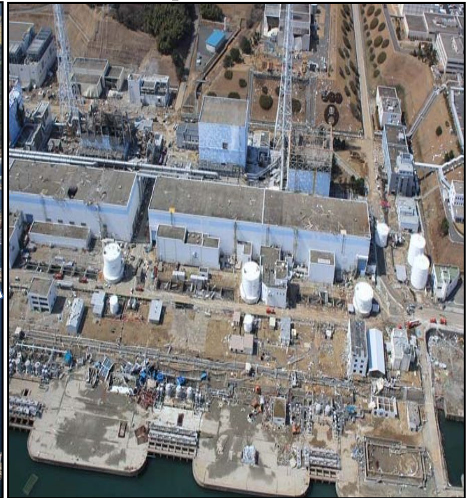
After the Earthquakes and Tsunamis
